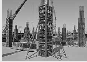
Column formwork
