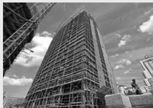
Working scaffolds façade
