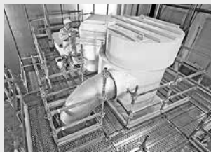
Working scaffolds industry
