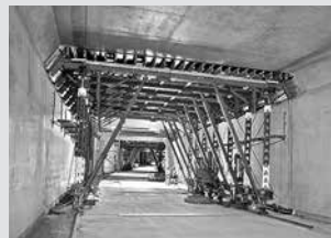
Tunnel Formwork
