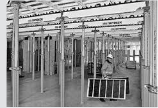
Slab Formwork
