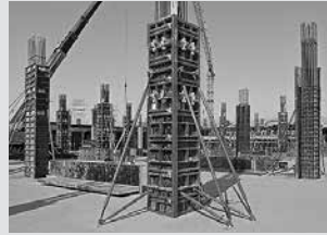
Column Formwork
