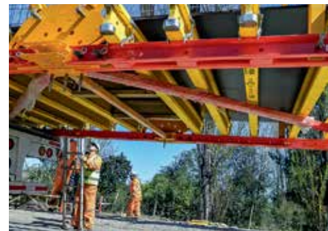
In addition to the usual VARIO Wall Formwork components, PERI UP components can also be used for the decking.
