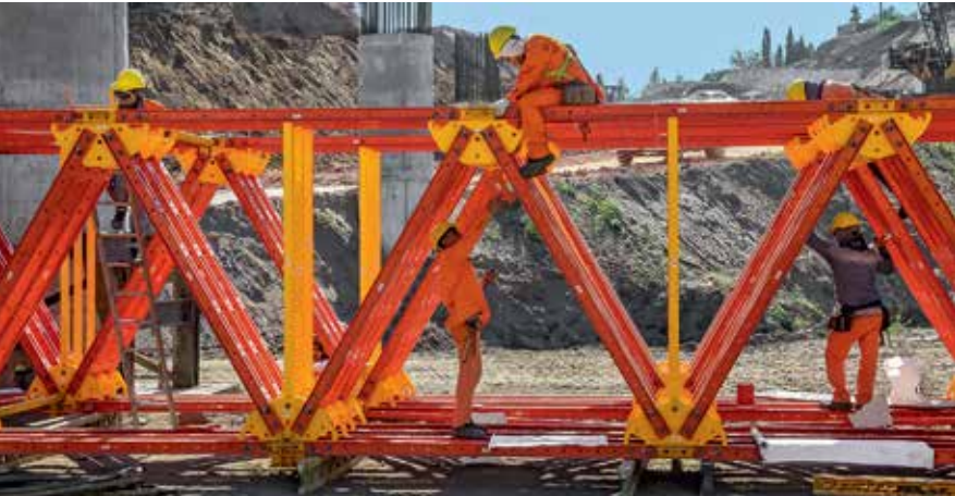
ALPHAKIT can be pre-assembled on the ground by hand without any crane assistance – only a minimum of space is required. As a result, the shoring system is also suitable for use on construction sites with limited space for assembly operations.
