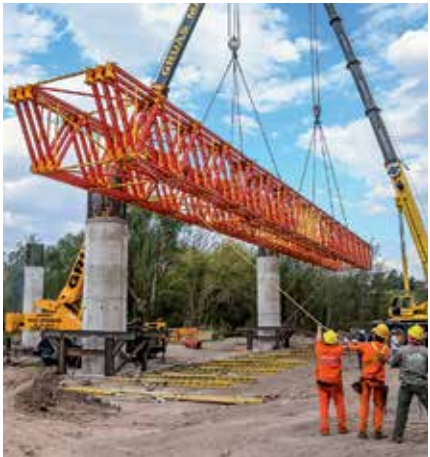
The lightweight towers and girder packages do not have to be split into multiple units for lifting purposes.
