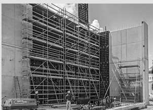
Working scaffold construction
