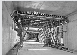
Tunnel formwork
