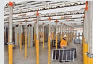
Slab Formwork
