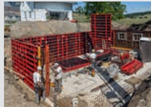
Wall Formwork
