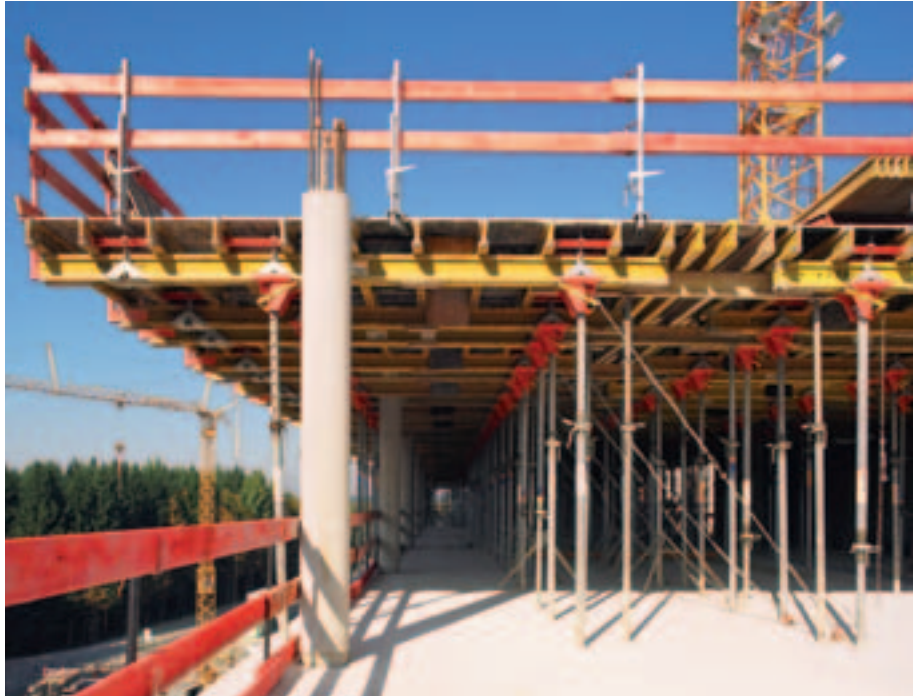
Cantilevering Table Modules VT. The anchoring chain is clearly shown here.
