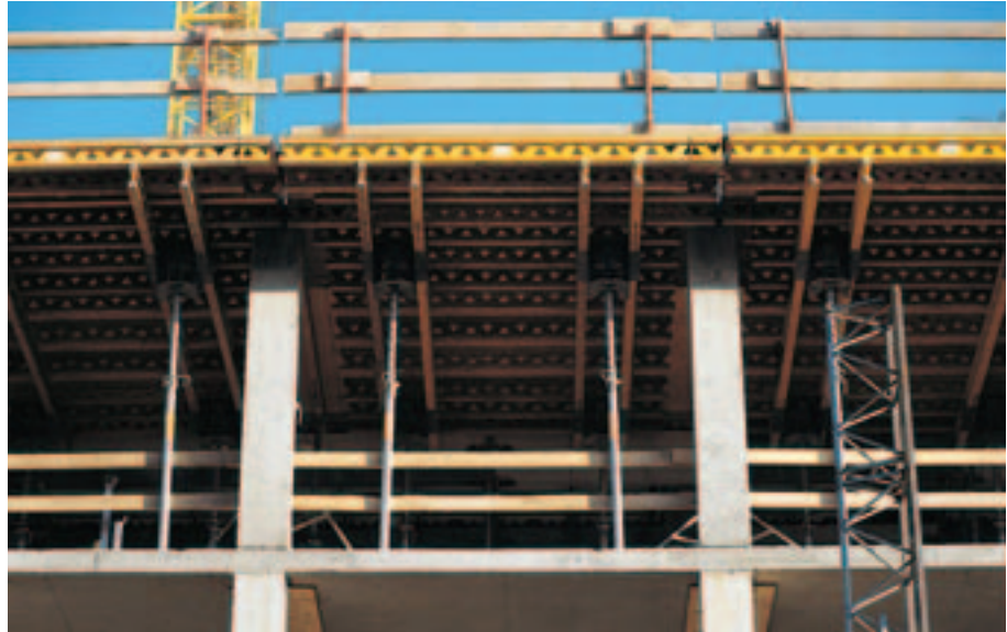
Safety guardrail system with PD 8 Guardrail Post, Item no. 019040.
