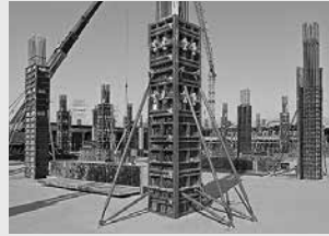
Column Formwork
