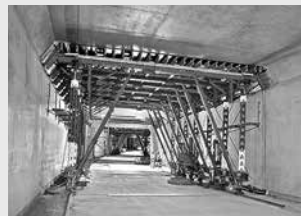
Tunnel Formwork
