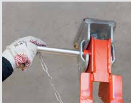
Step 5 Fixing the VGK with bolts
