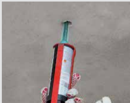
Step 2 Injecting the composite mortar
