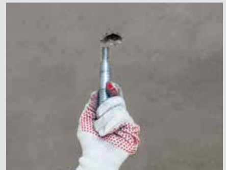
After dismantling the bracket Removing the re-usable Anchor Bolt
