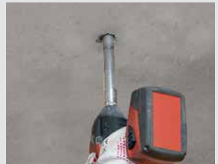
Step 3 Screwing in the refurbishment anchor by means of an impact wrench
