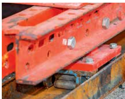
The cantilevered parapet carriage being moved on a heavy-duty roller.
