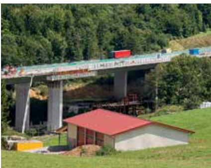
During the bridge construction work, traffic on the A 81 motorway was able to use the already completed superstructure between the Geisingen and Engen junctions.
